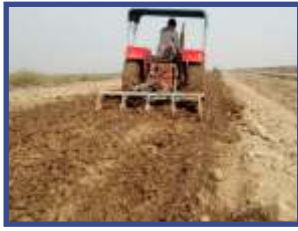
Scarifying The Surface
